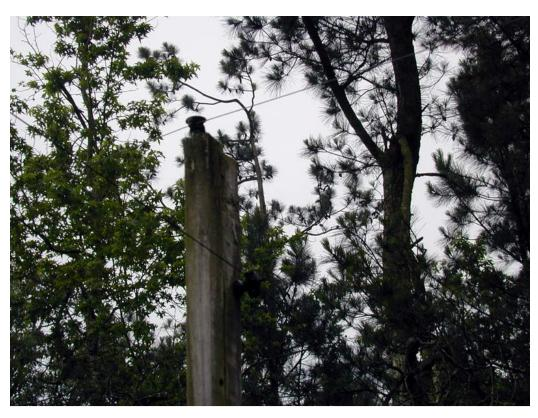
For end supports, I use trees, pressure treated lumber, or landscaping timbers. With a lot of tension, I backstay the poles to a dead-man (generally an old brick) buried in the ground. When I set end-posts with my power auger, I line the hole with copper flashing. That becomes part or all of the feed point (and termination) ground connection.
